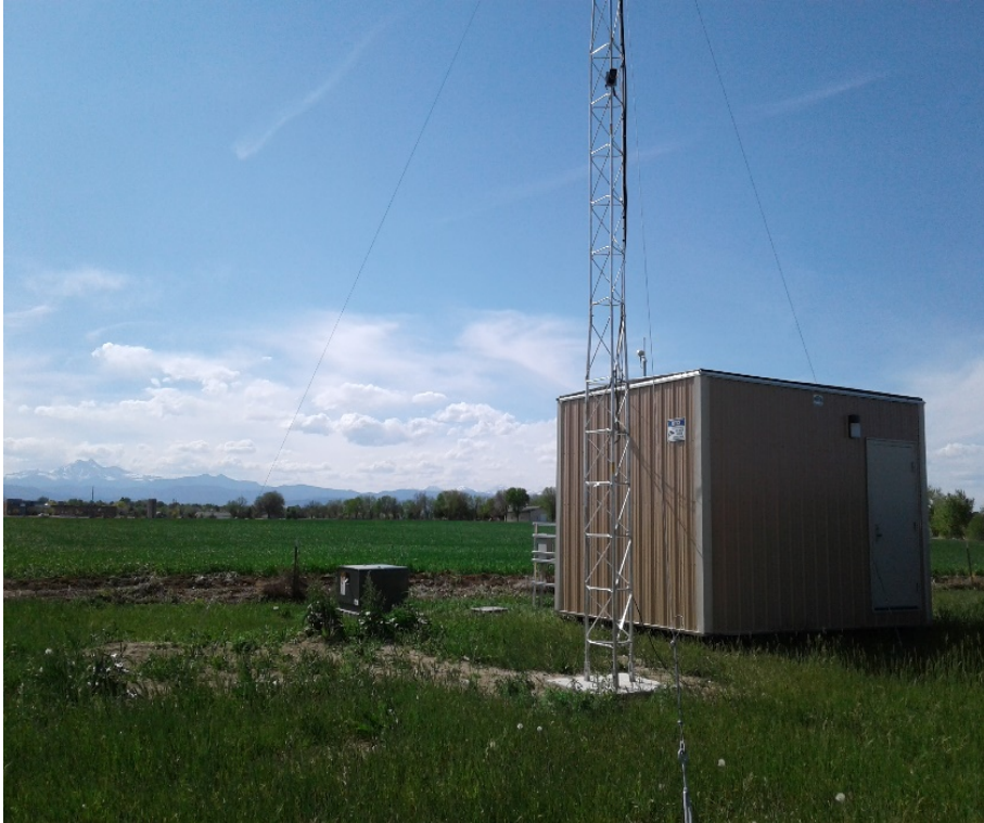
LUR instrument shelter with adjacent meteorological tower
